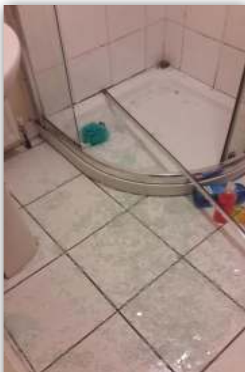
Glass on bathroom floor: unresolved faulty shower door
