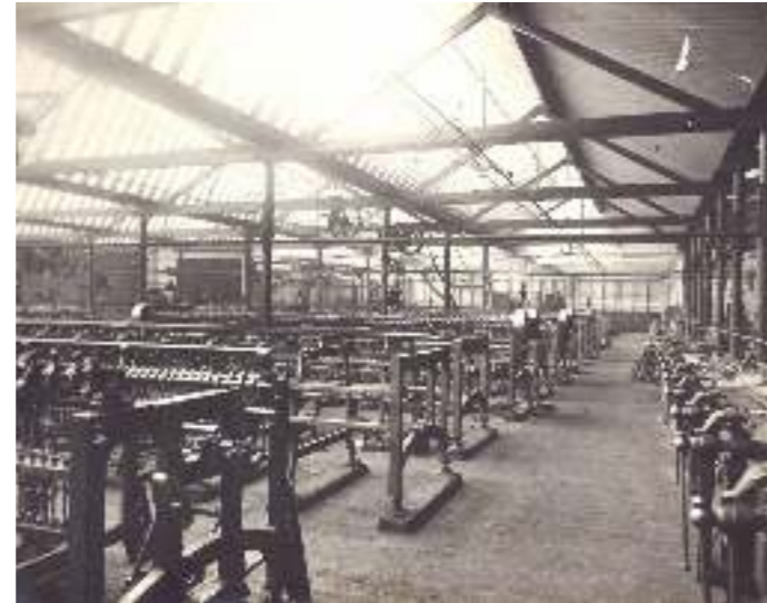
Old Mackies Site - Internal factory view
