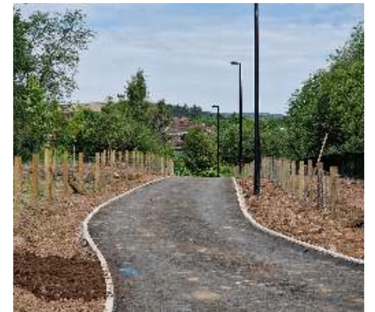
Existing greenway works
