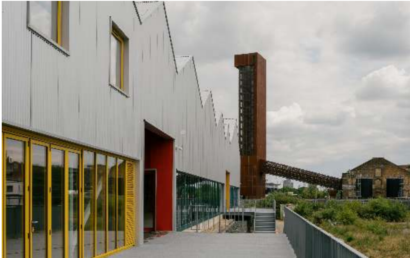
Turner Works - Hackney Bridge
