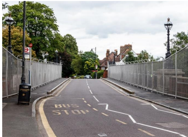
Figure 2 Archway Bridge's anti-suicide fencing (WHPARA, 2019)
