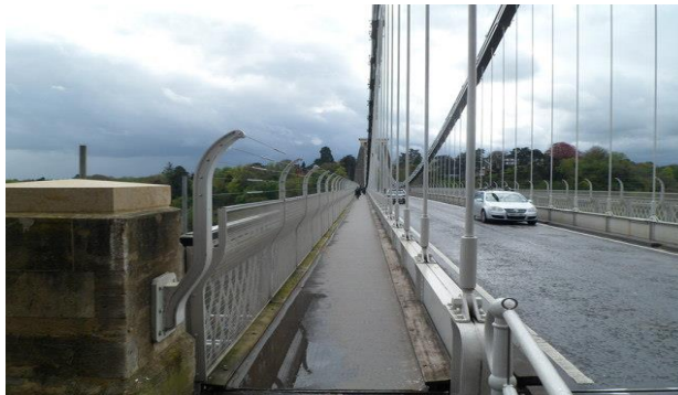
Figure 3 Barriers along the Clifton Suspension Bridge, Bristol (Jaggery 2012)
