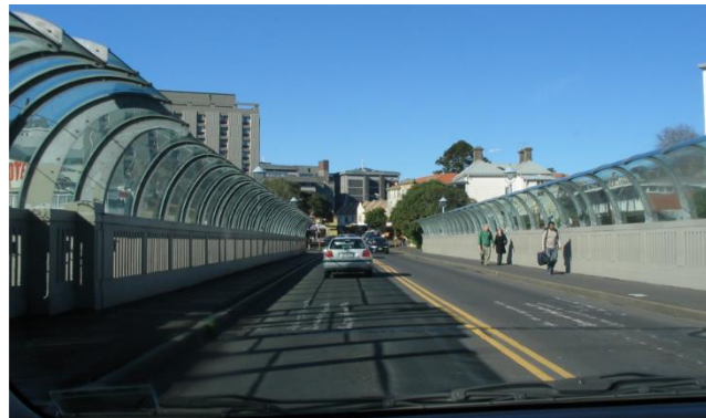
Figure 6 Current barrier system on the Grafton Bridge
